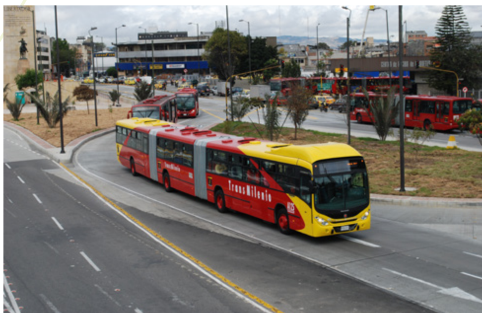
Bogotá BRT System (Transmilenio)
