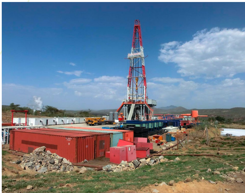
KenGen geothermal drilling rig, Olkaria, Kenya
